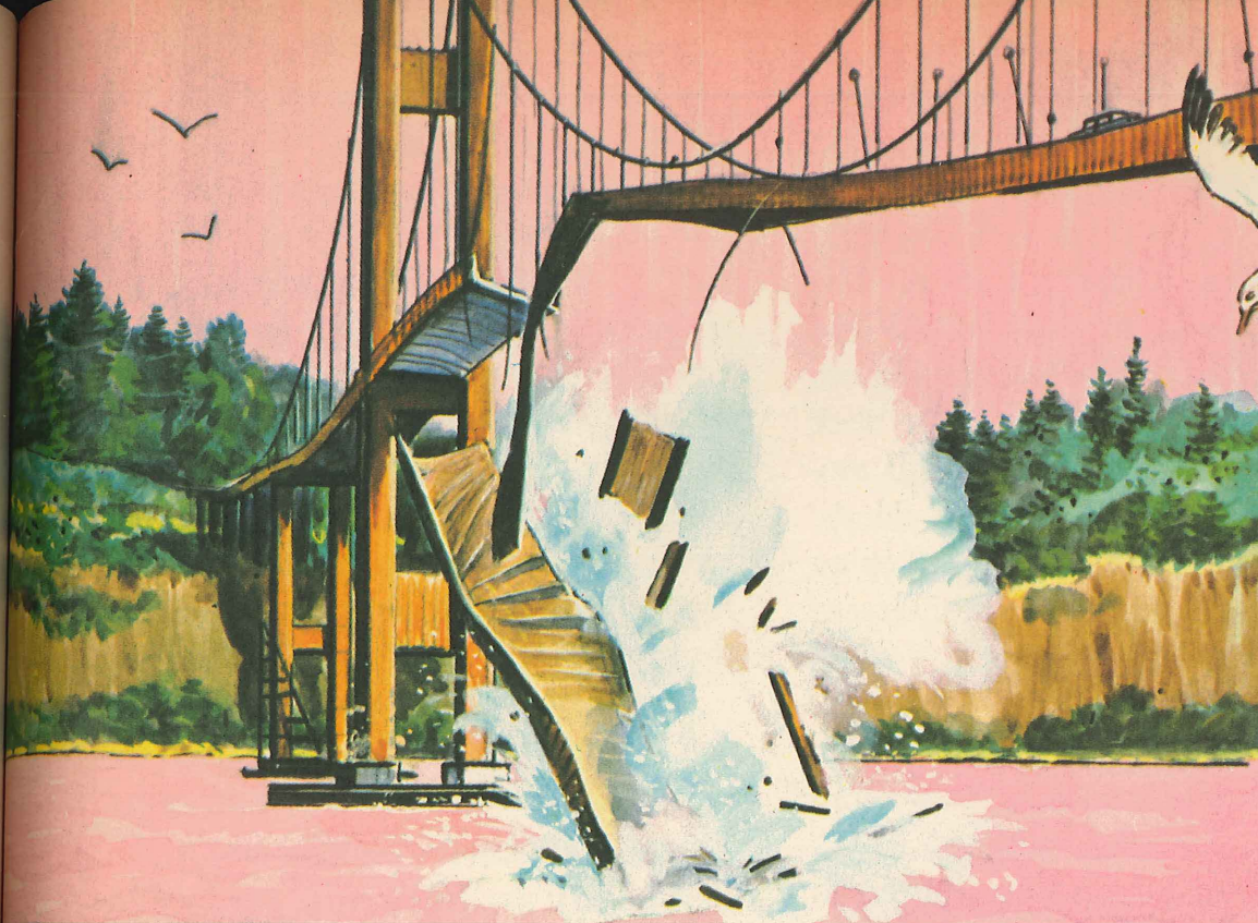
On November 7, 1940, a wind of over 35 miles an hour made the Tacoma Narrows Bridge in Washington swing and twist. Only four months after its completion, the structure was destroyed.
